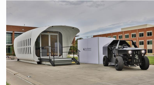
ORNL 3D printed house & utility vehicle
